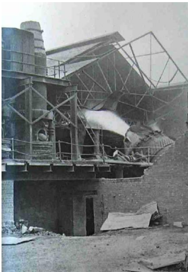
Figure 4.1- A Bessemer Converter during a ‘Bessemer blow’ at the Glengarnock Steelworks. This photograph is not dated, but would have been taken between 1885 and 1920, when these furnaces were in operation here. Image from Glengarnock | Clydebridge (cfindlay17.wixsite.com) .
