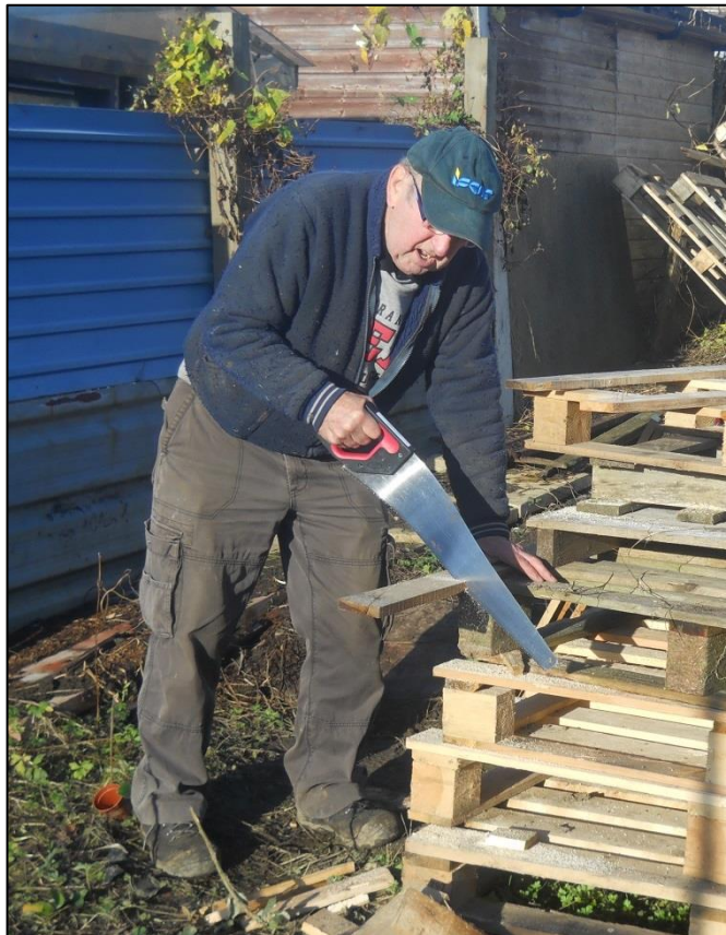
Figure 4: Harry building a shed for a new plotheholder from wooden pallets (Image: By author)
