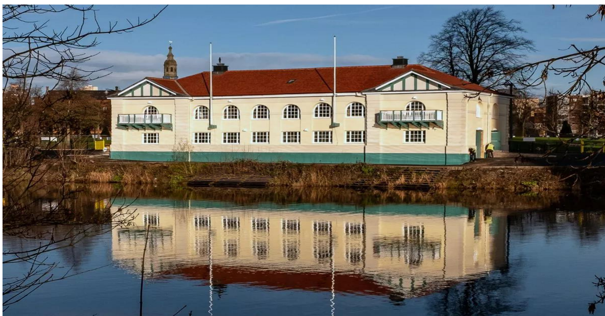
Figure 22. Renovated West Boathouse
