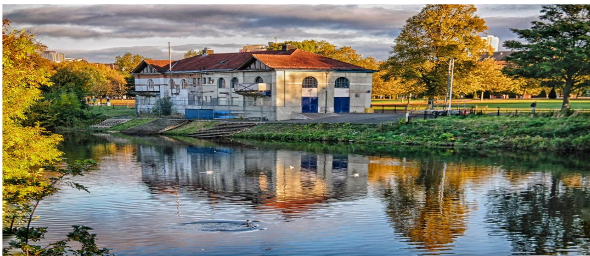
Figure 20. West Boathouse before renovation.
