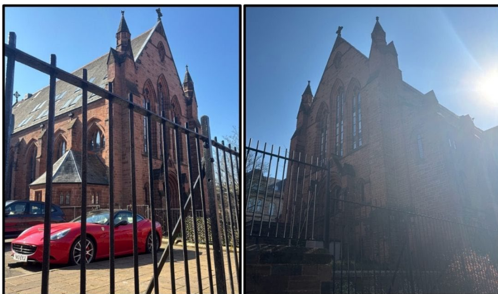
Figure 51 – Site of the Former Belmont Church
